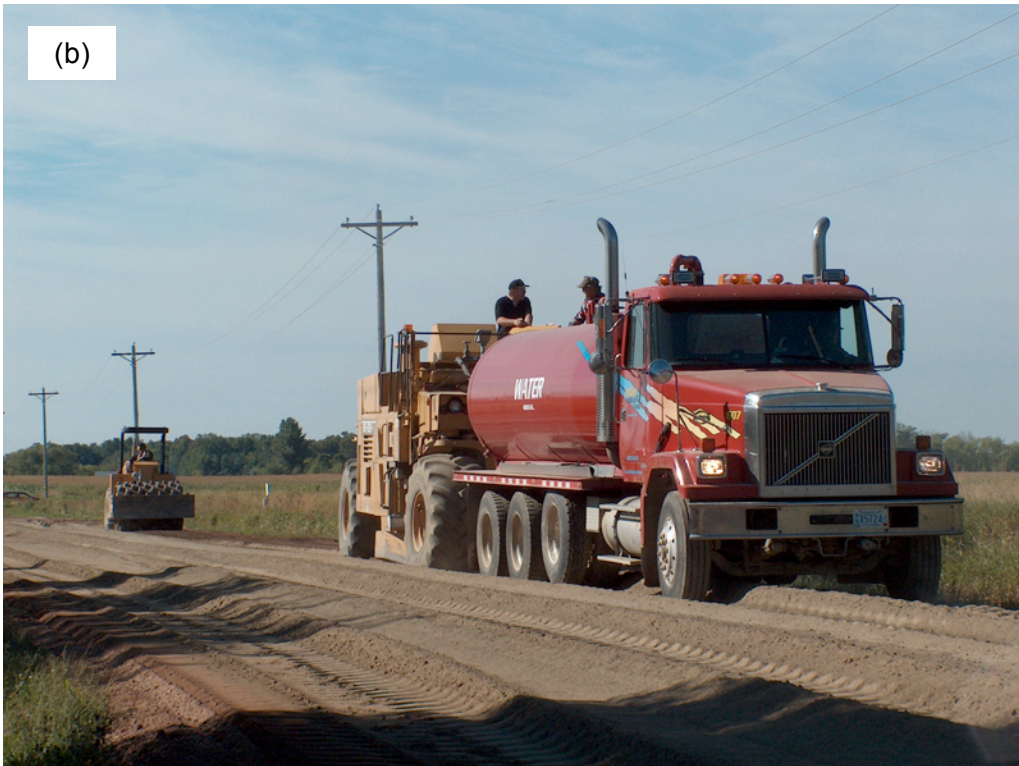
Fig. 2 (a) Spreading of fly ash on gravel road with lay-down equipment and (b) Mixing process of fly ash, road-surface gravel, and water by a reclaimer (compaction is performed right after mixing by tamp-foot compactor seen in the background).
