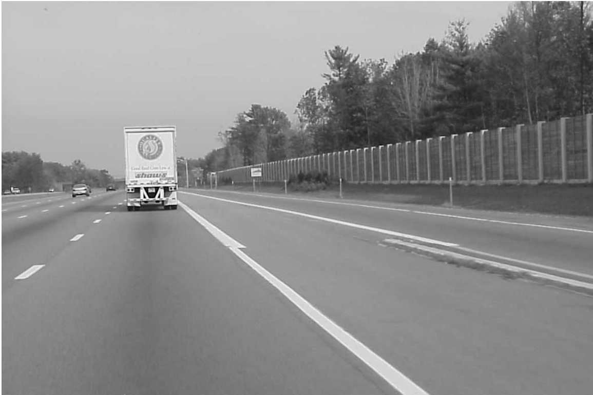
Figure 3 Noise barrier reducing noise entering residential community
