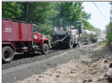
Reclaimer pushing the asphalt tanker and introducing the foamed asphalt into the base.
