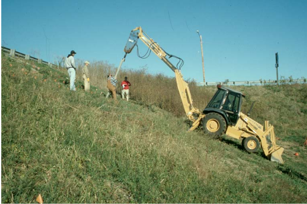
Figure 3.11 Initial equipment used for installation of RPPs at the I70-Emma slide 1.
