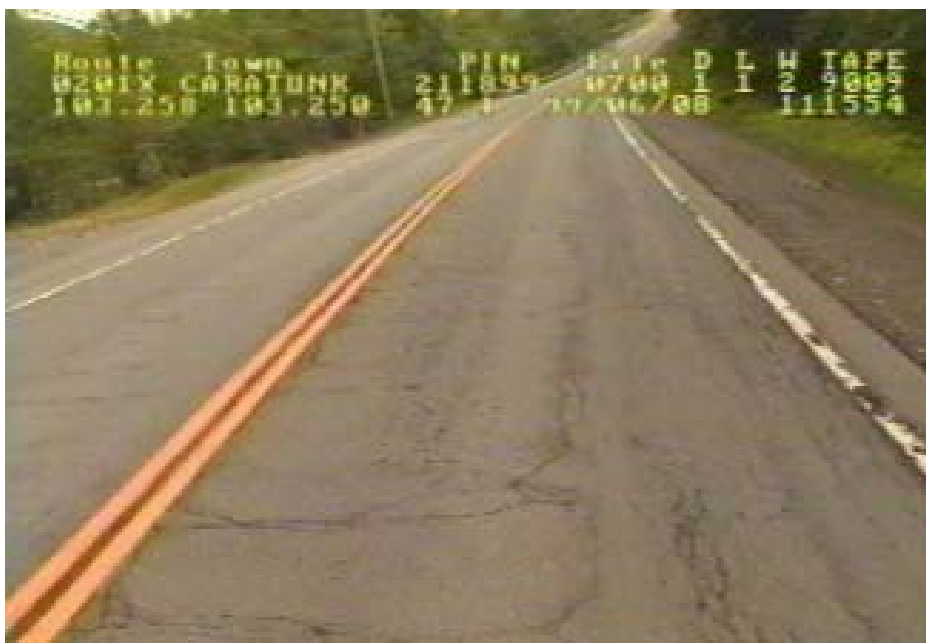
FIGURE 4.1 Photo of typical section
