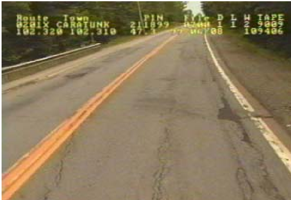
FIGURE 4.2 Photo of typical section
