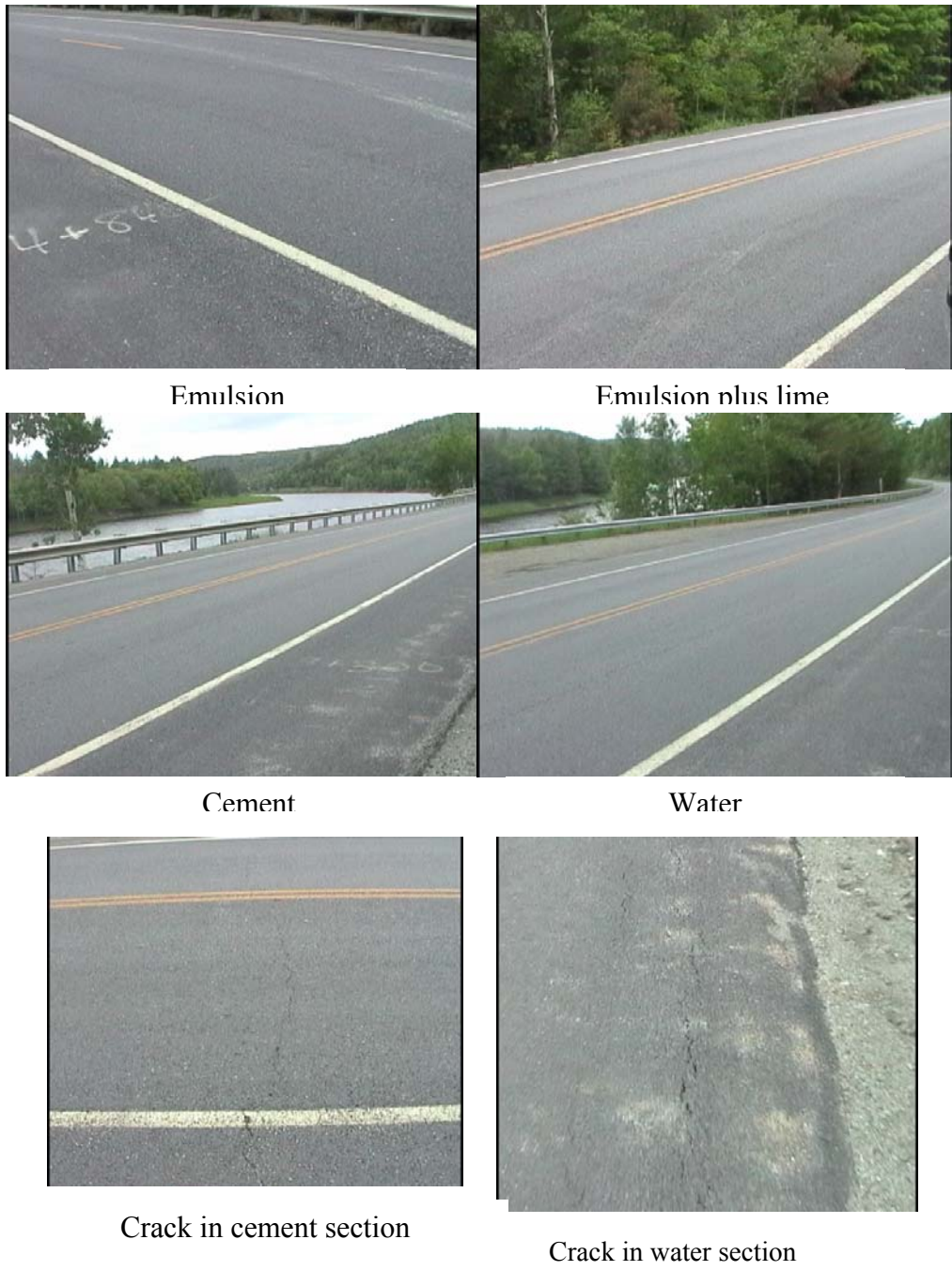
FIGURE 16.1 Photos of recycled sections after one year of construction
