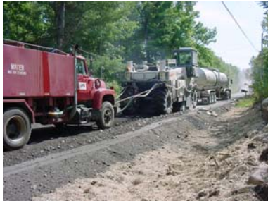
Figure 7. Foamed Asphalt Full Depth Reclamation Construction
