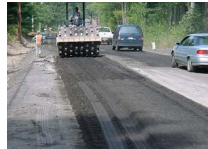
Figure 8 Compaction of Full Depth Reclamation Layer
