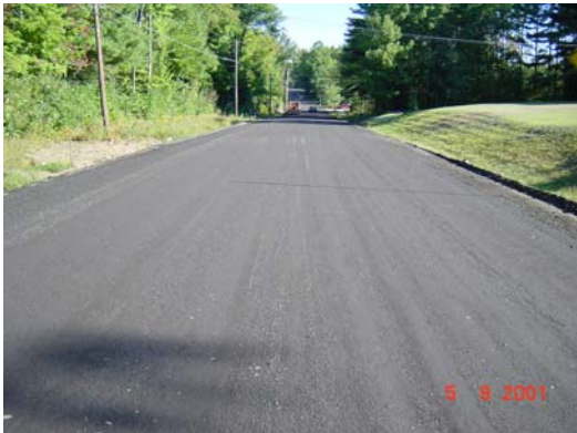
Figure 9. Completed Foamed Asphalt Layer
